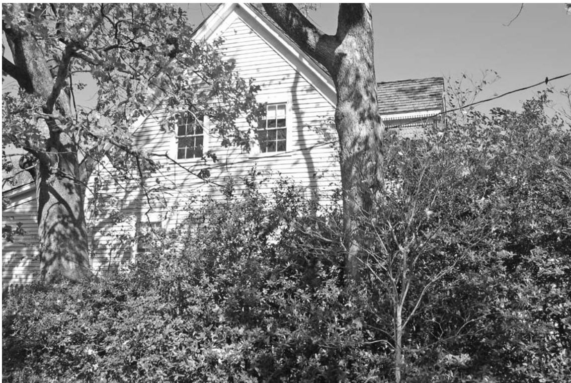
Photograph 7: View looking at the left side elevation of the resource.
