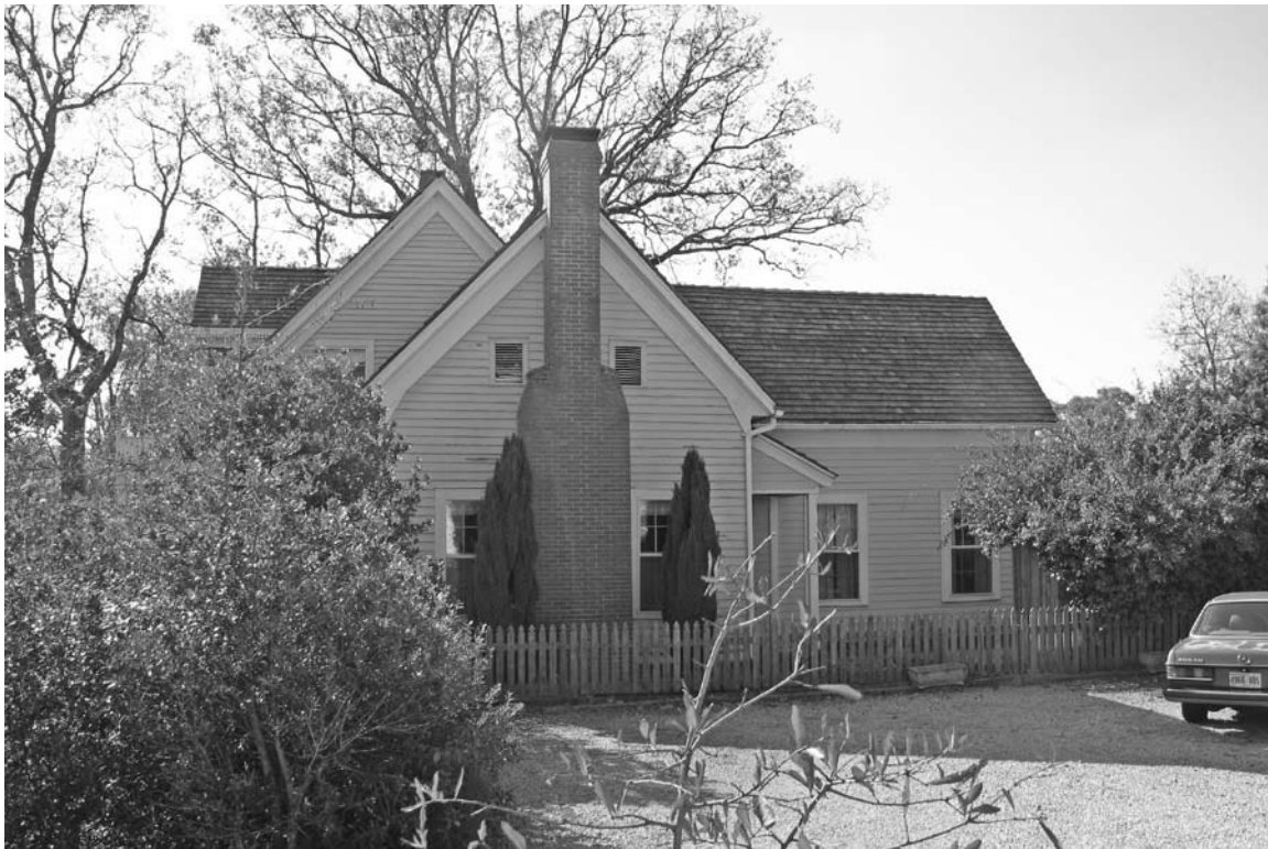
Photograph 1: View of the right elevation of the resource.
