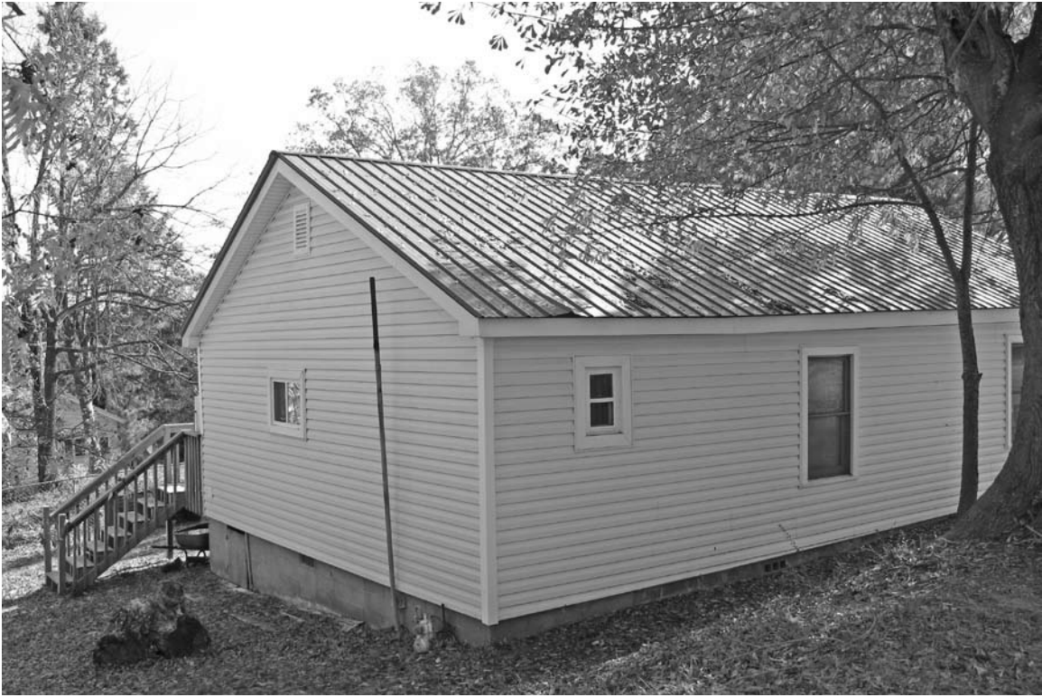
Photograph 3: View looking at the rear and left side elevation of the resource.
