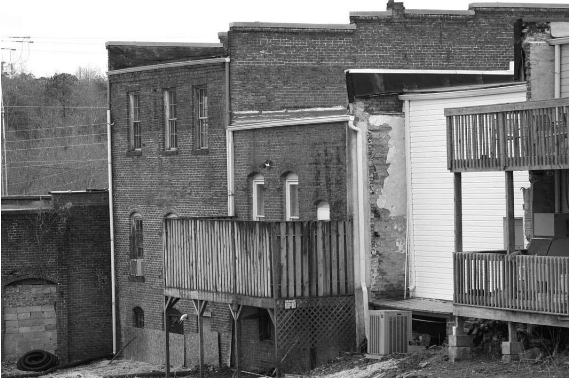
Photograph 2: Rear elevation of the resource.
