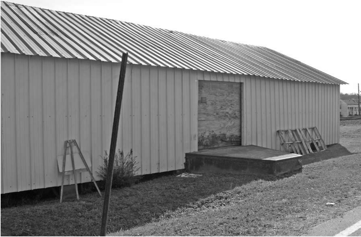
Photograph 1: View of the front elevation of the resource.
