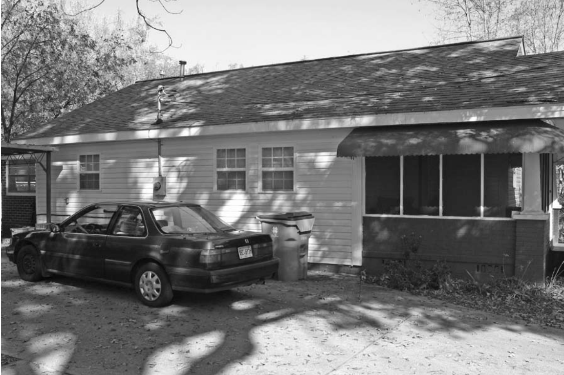
Photograph 2: Left side elevation of the resource.
