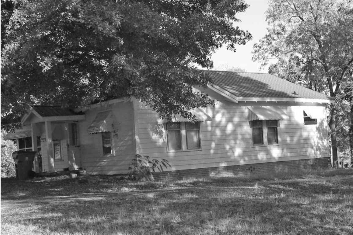
Photograph 2: Right side elevation of the resource.
