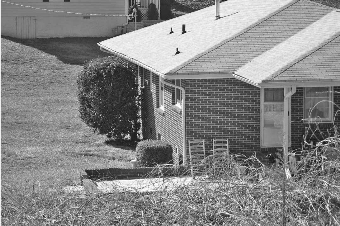
Photograph 4: View looking at the rear elevation of the resource.
