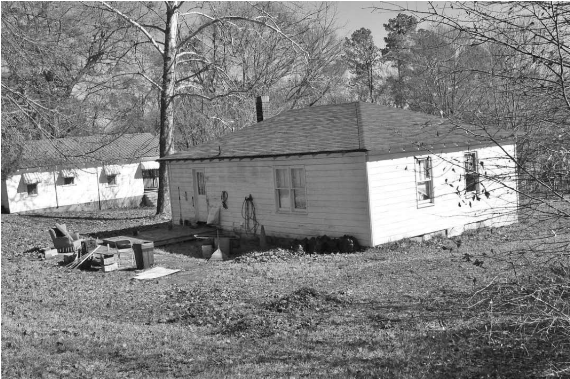
Photograph 3: View looking at the rear elevation of the resource.
