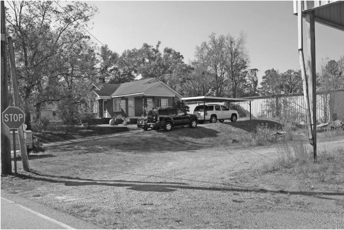
Photograph 1: View looking at the right side elevation of the resource.
