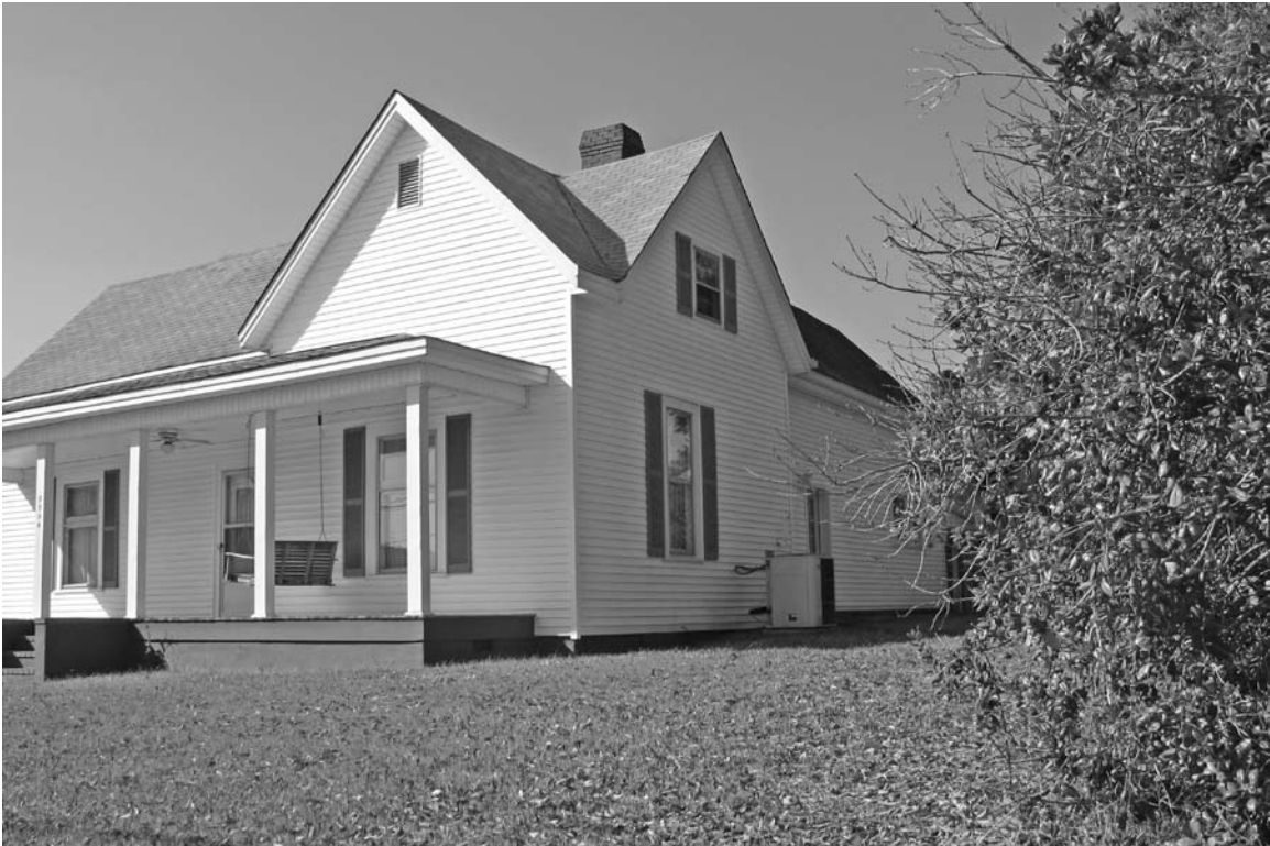
Photograph 1: Front and right side elevation of the resource.
