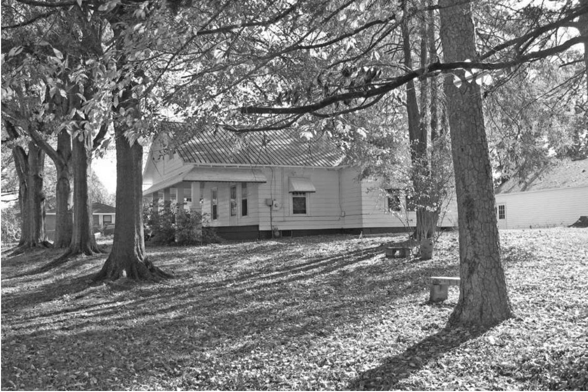
Photograph 1: View looking right side elevation the resource.
