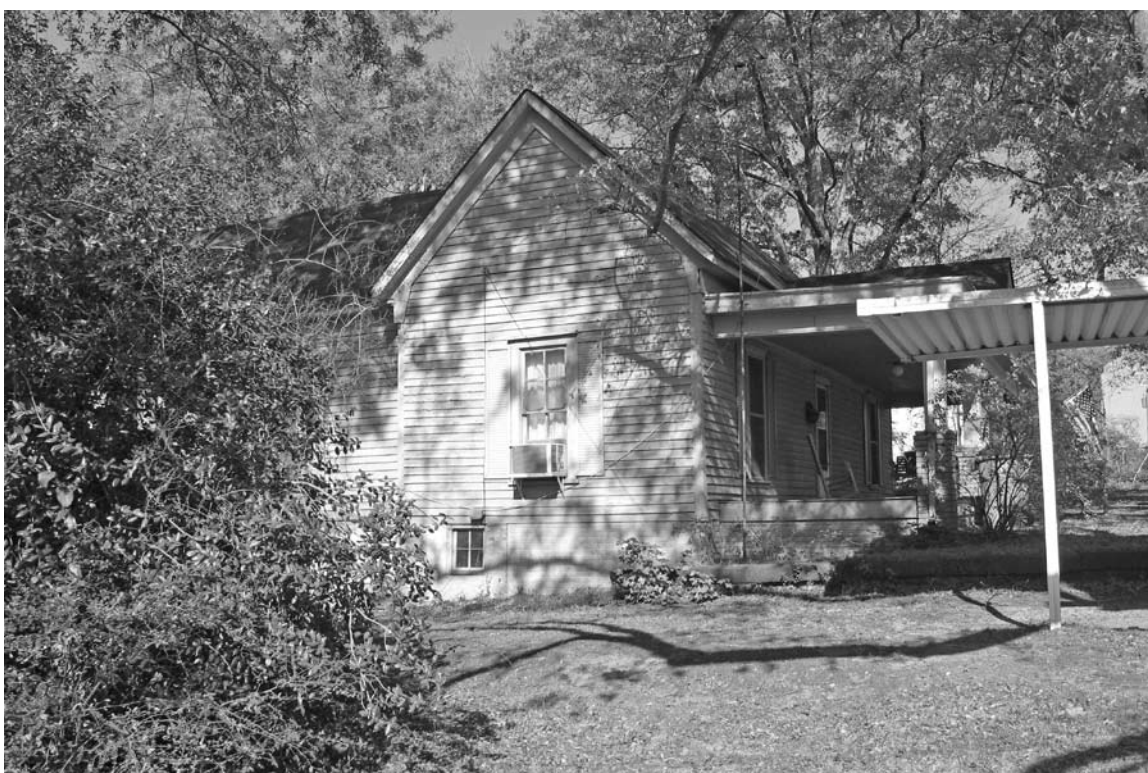
Photograph 2: View looking at the rear and left side elevation of the resource.
