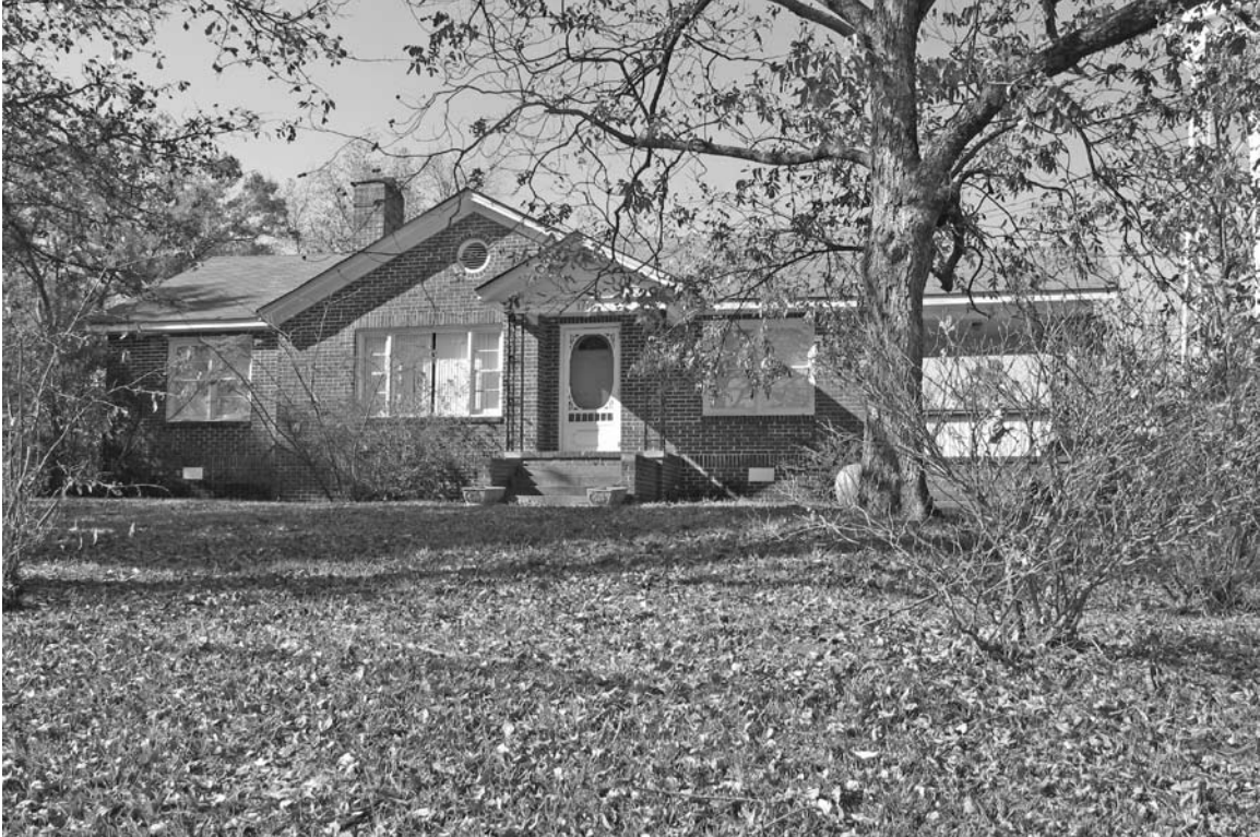
Photograph 2: View looking at the front elevation the resource.
