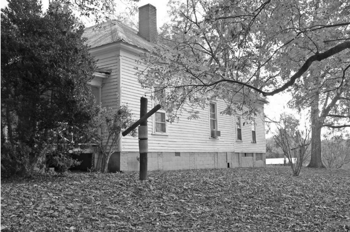
Photograph 6: View looking at the right side elevation of the resource.
