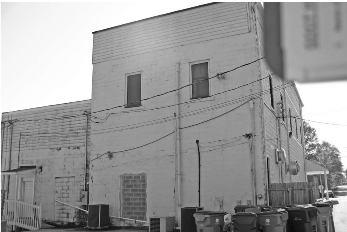
Photograph 6: View looking at the rear elevation of the resource.
