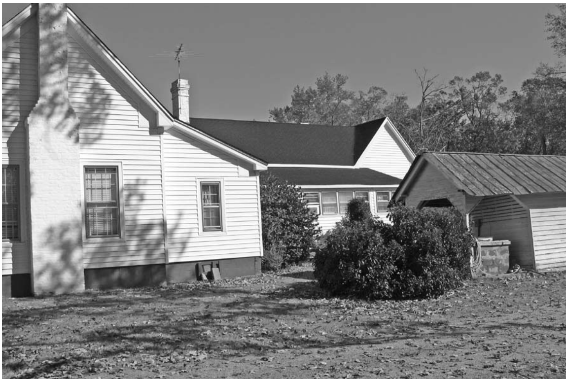
Photograph 7: View looking at the rear elevation of the resource.
