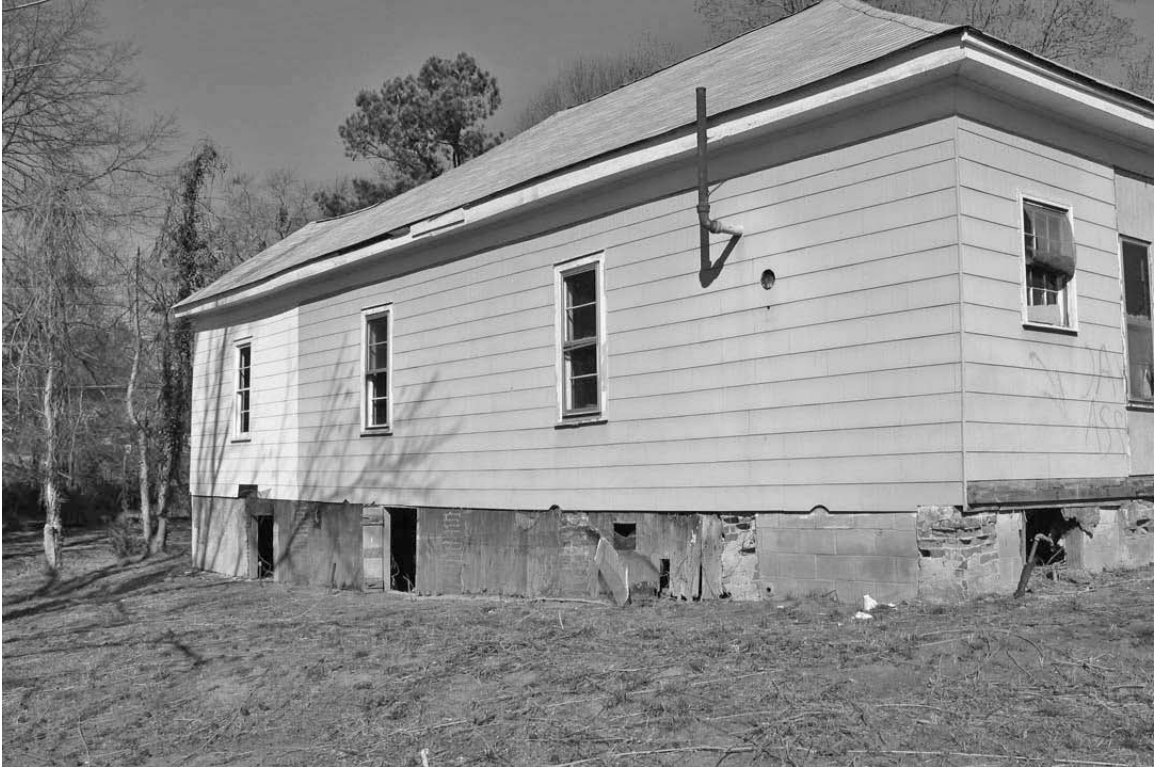
Photograph 4: View looking at the right side elevation of the resource.
