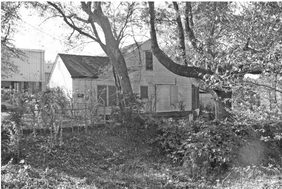
Photograph 1: View of the rear elevation of the resource.
