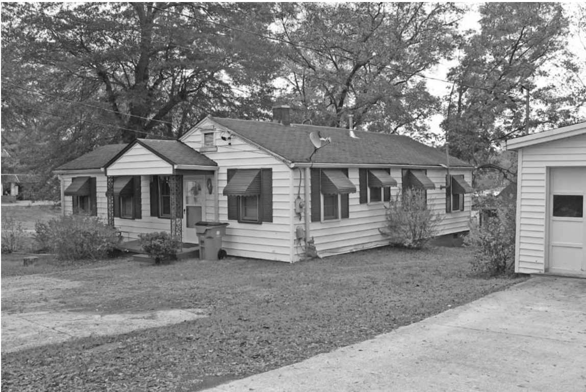
Photograph 7: View looking at the right side elevation of the resource.
