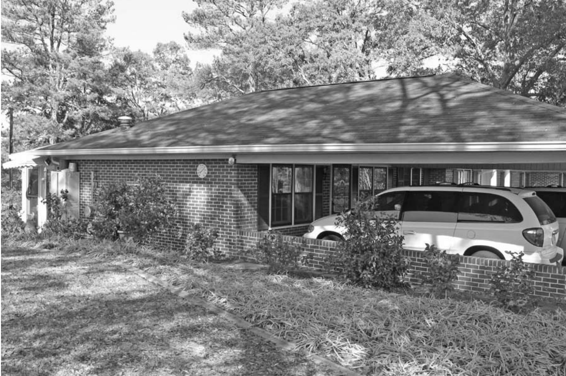
Photograph 2: View of left side elevation of the resource.
