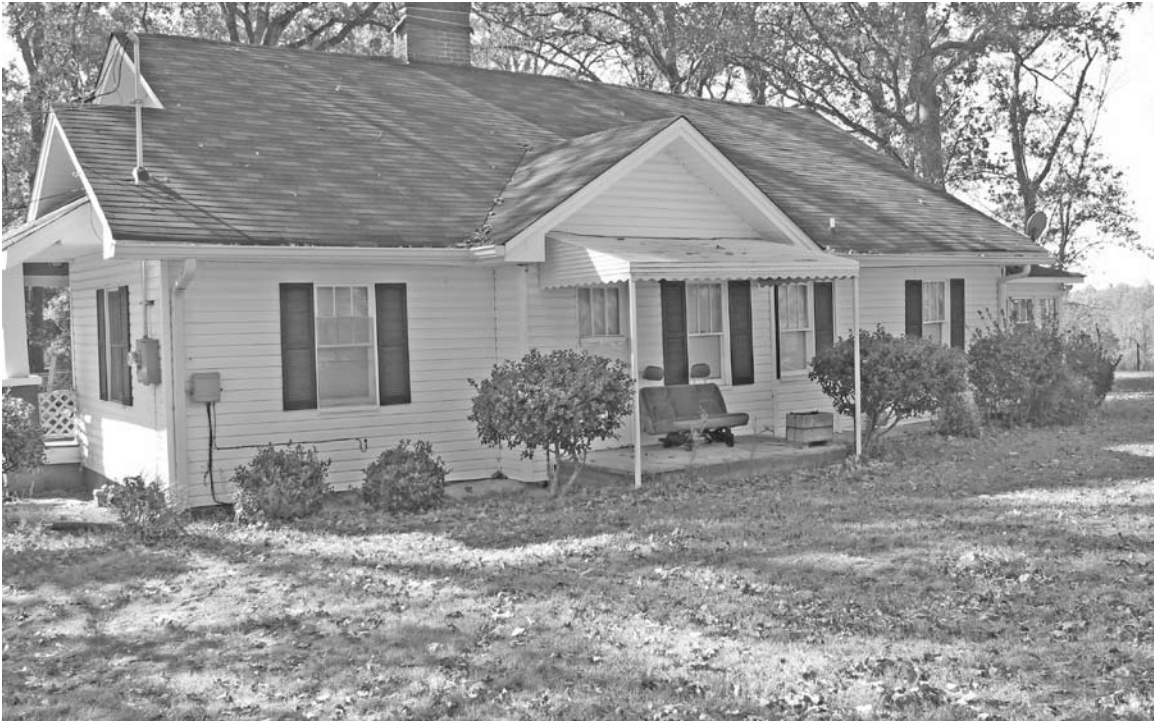
Photograph 3: View of the rear elevation of the resource.
