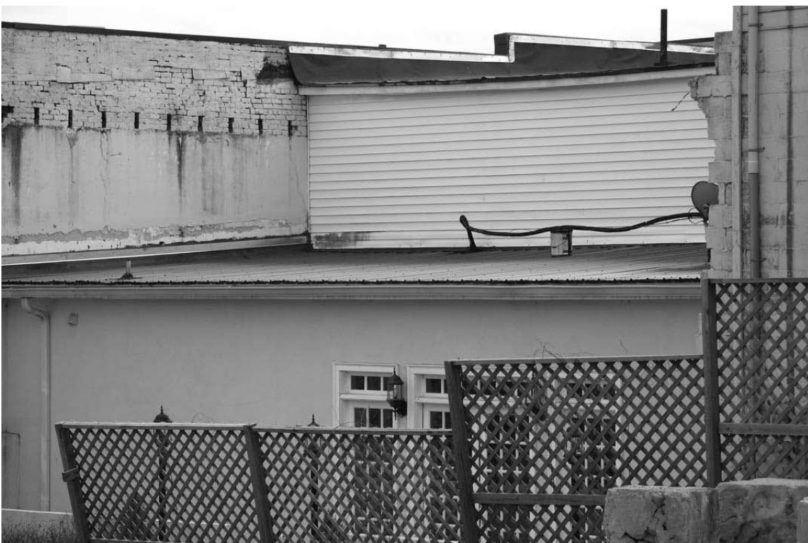
Photograph 2: Rear elevation of the resource.
