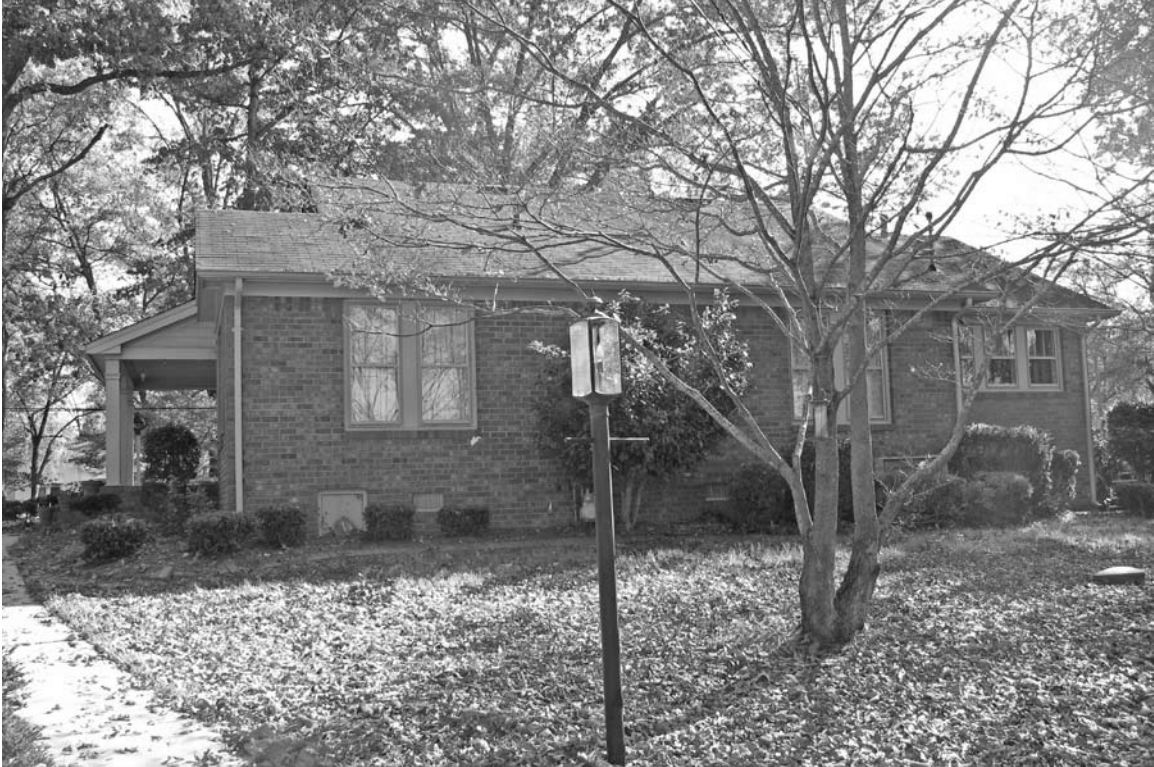
Photograph 2: Right side elevation of the resource.
