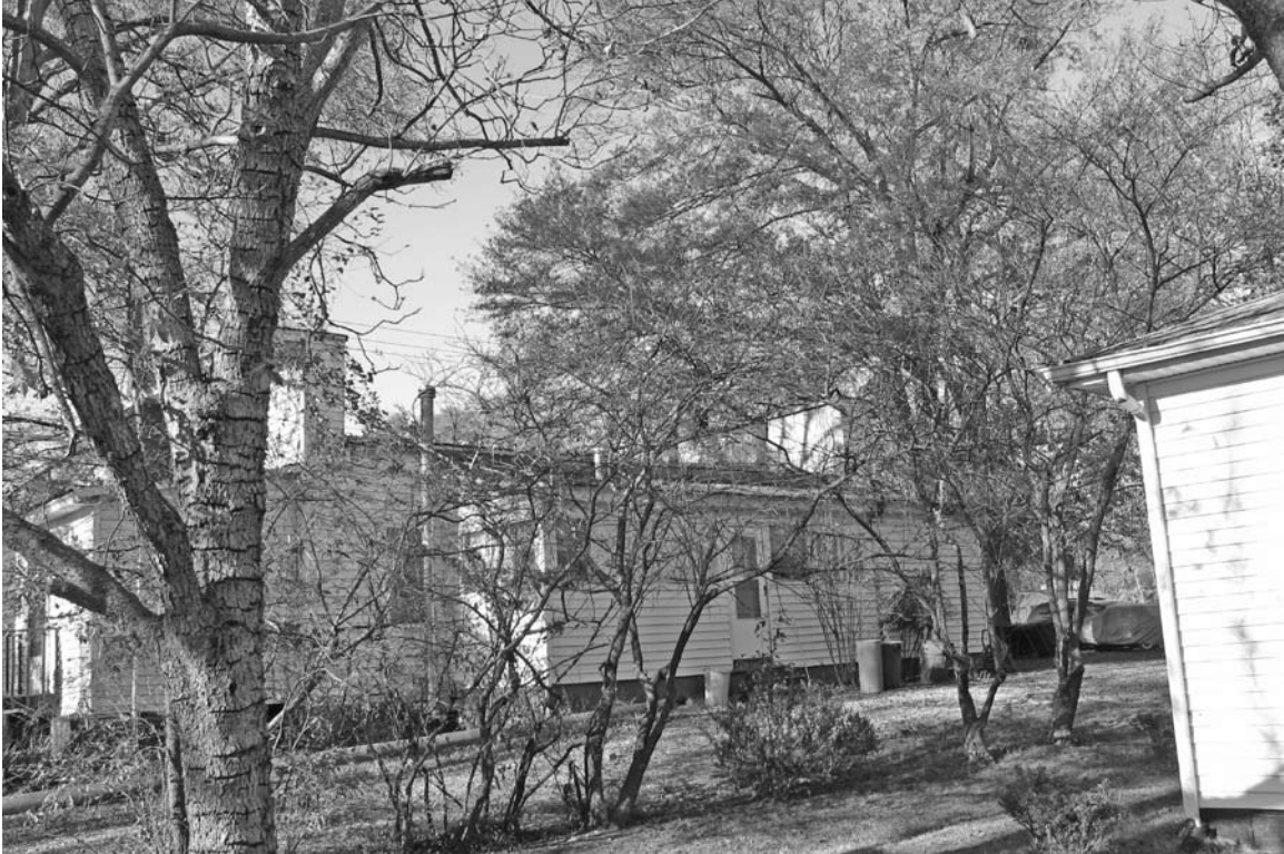
Photograph 4: View of the rear elevation of the resource.
