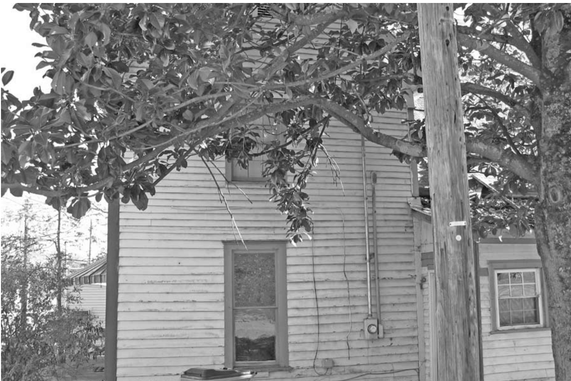
Photograph 2: View looking at the right side elevation of the resource.
