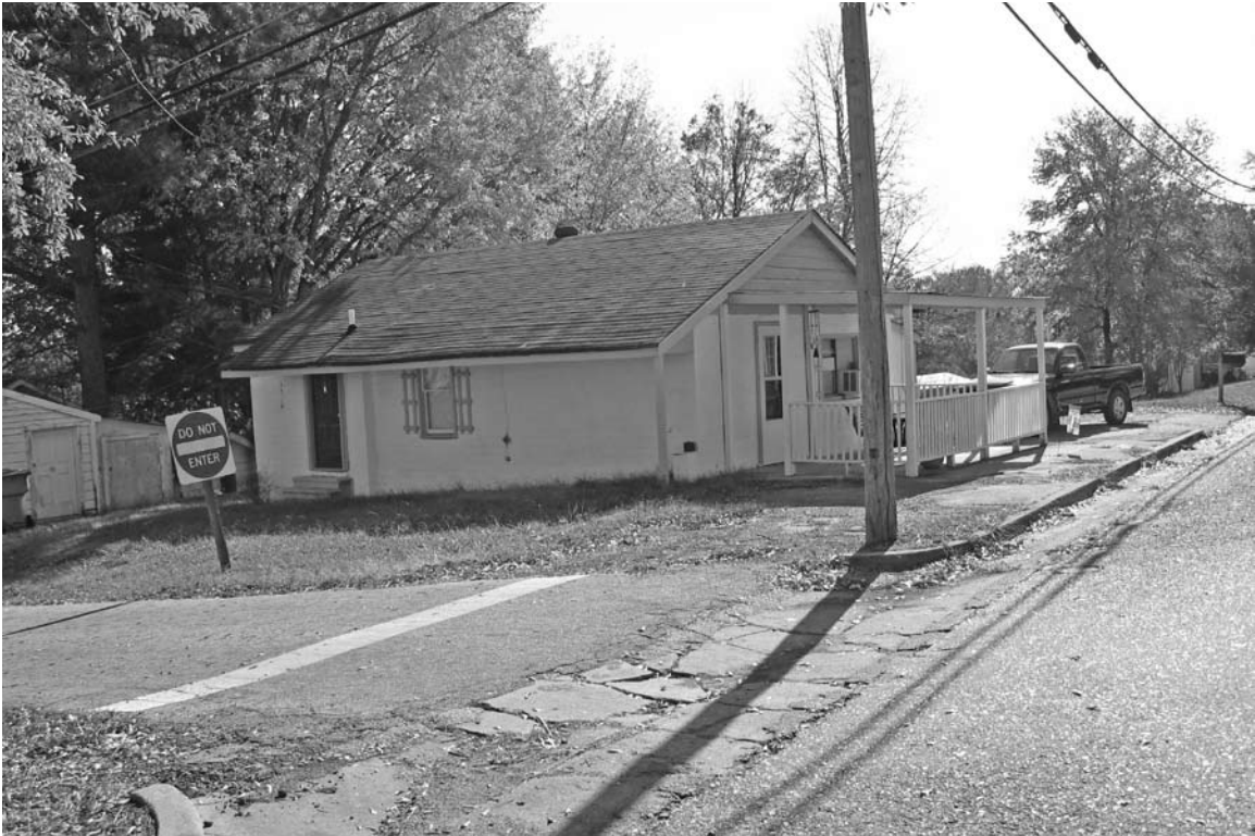
Photograph 1: View looking at the left side elevation of the resource.
