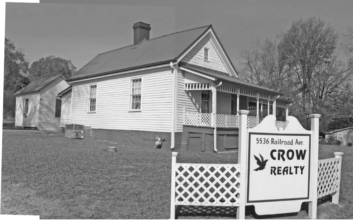
Photograph 3: View looking at the left side elevation of the resource.
