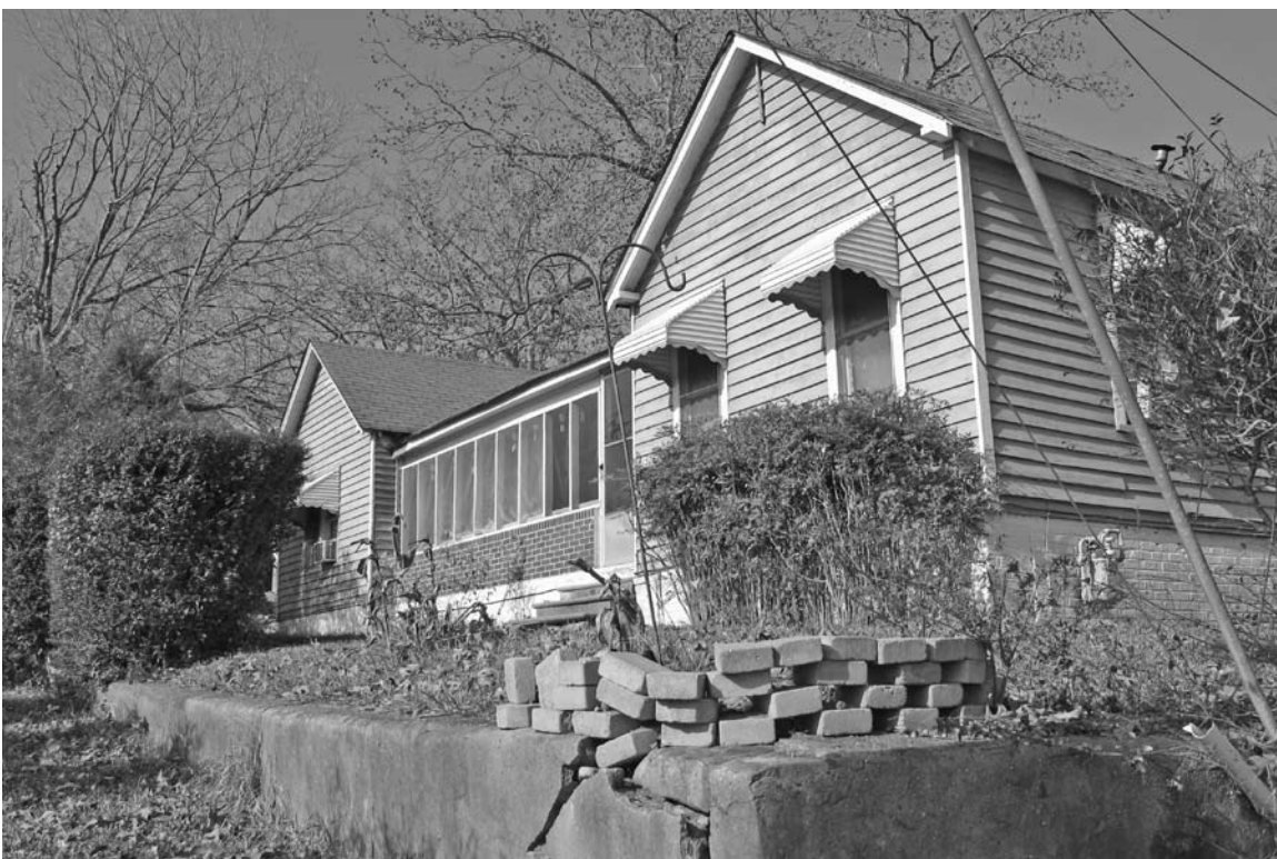
Photograph 2: View looking at the front portion of the right side elevation.
