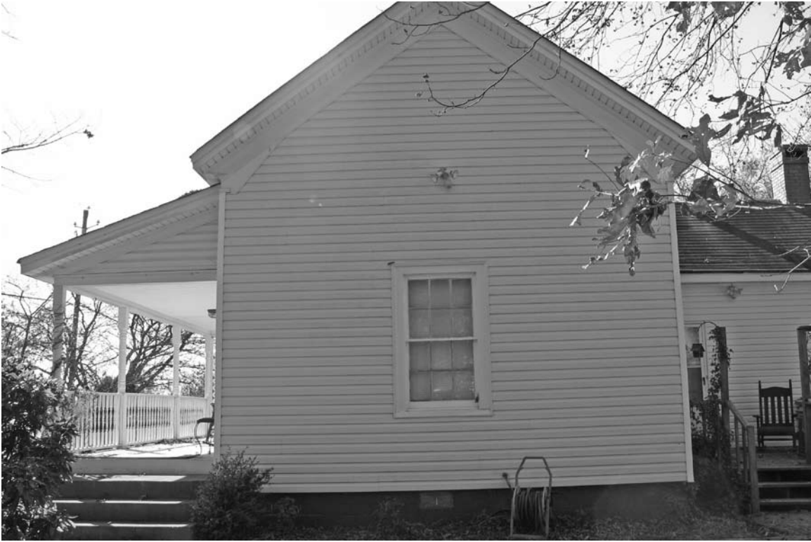
Photograph 3: View looking at right side elevation of the resource.
