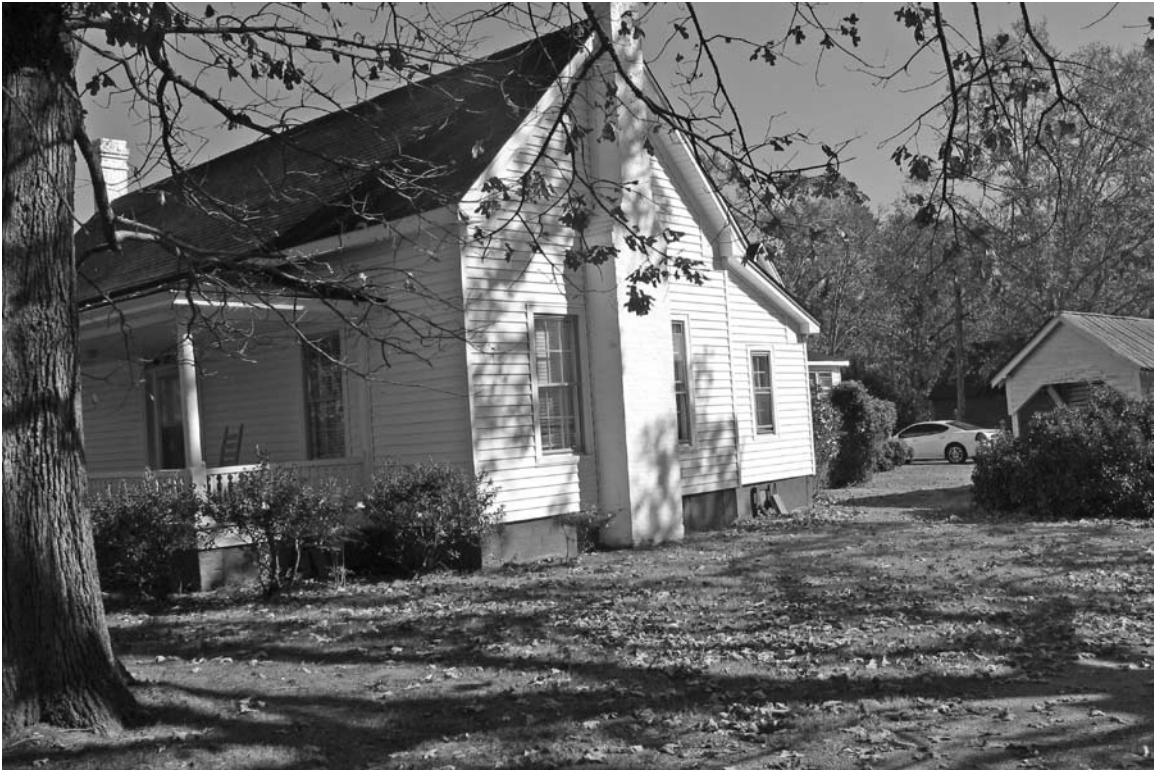
Photograph 5: View looking at the right side elevation of the resource.
