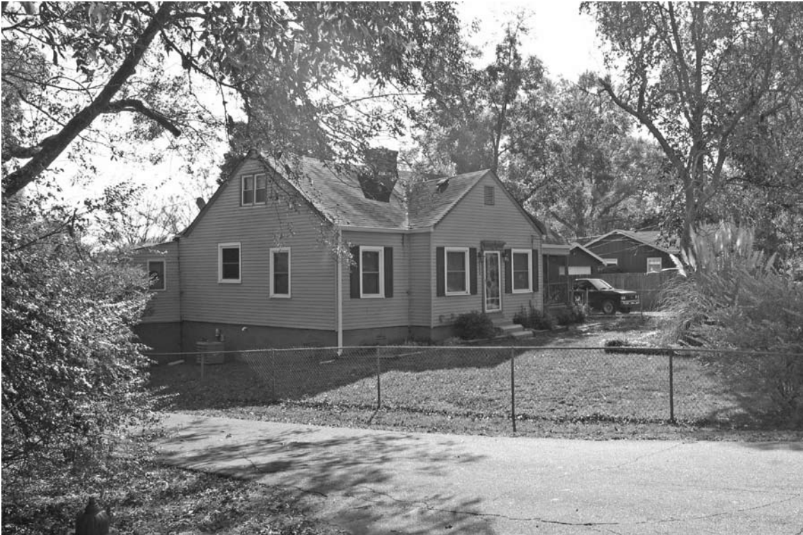
Photograph 1: View of left side elevation of the resource.
