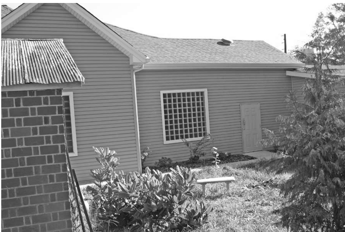
Photograph 2: View looking at the right side elevation the resource.
