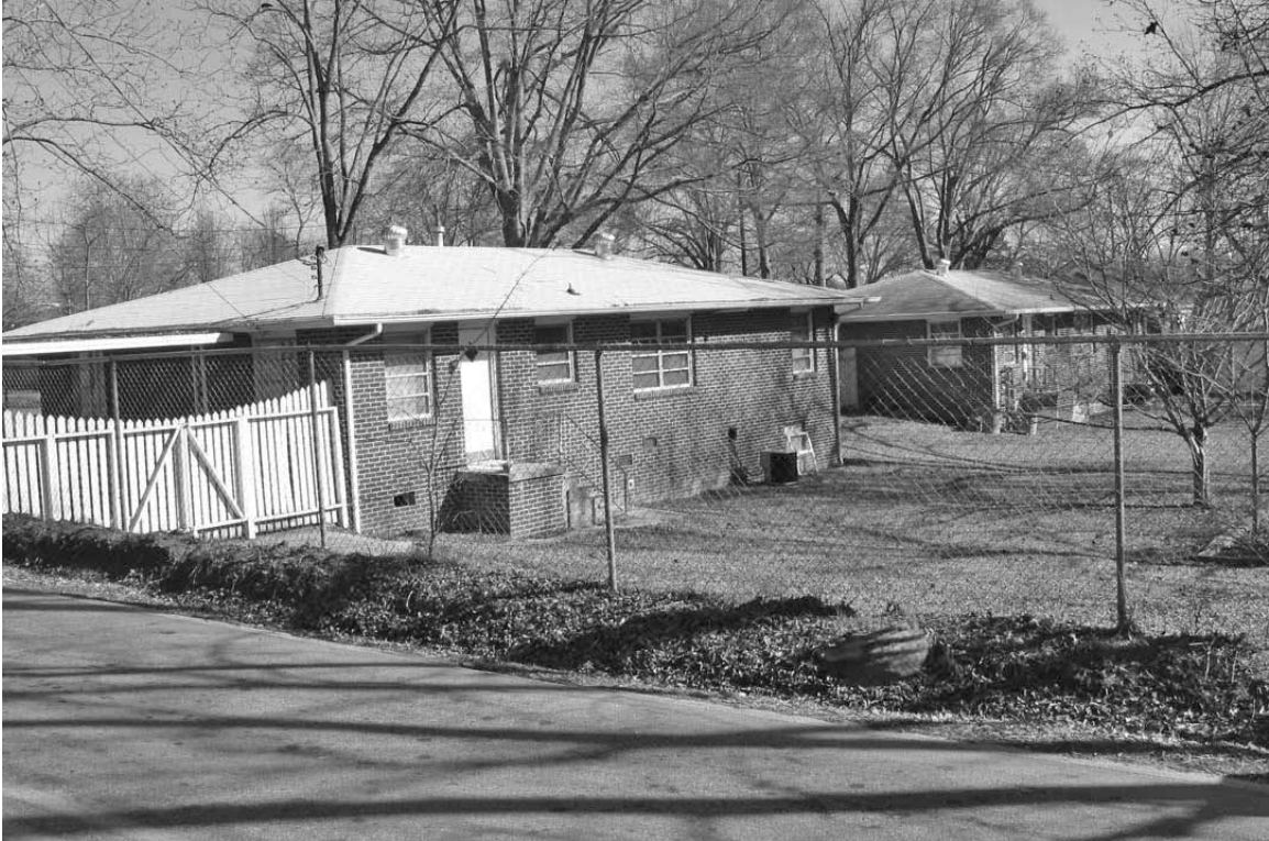
Photograph 2: View looking at the rear elevation of the resource.
