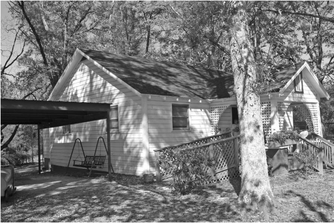
Photograph 3: View looking at the left elevation of the resource.
