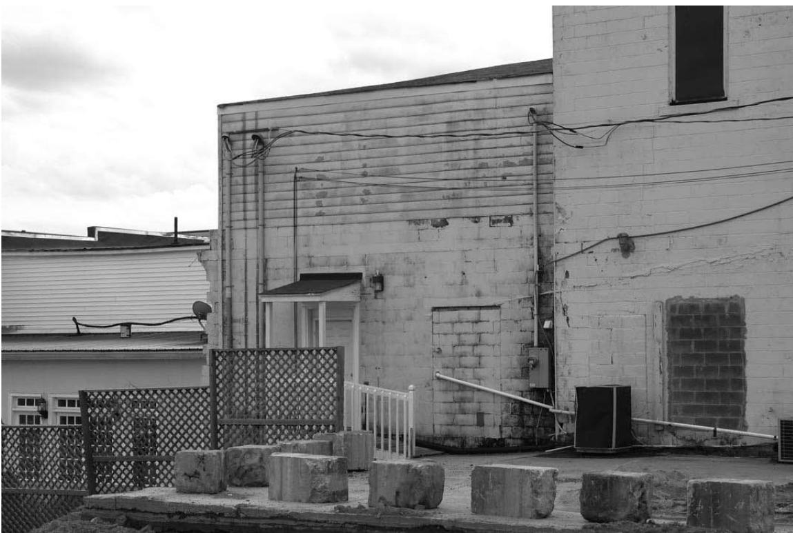
Photograph 4: Rear elevation of the resource.
