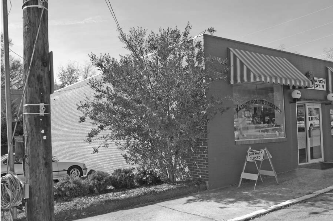
Photograph 2: View of left elevation of the resource.
