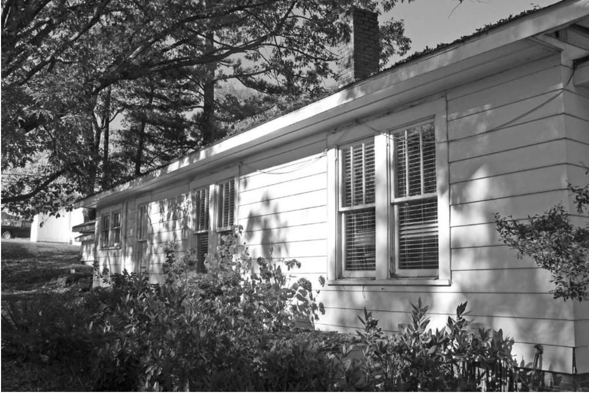
Photograph 5: View looking at the left side elevation of the resource.
