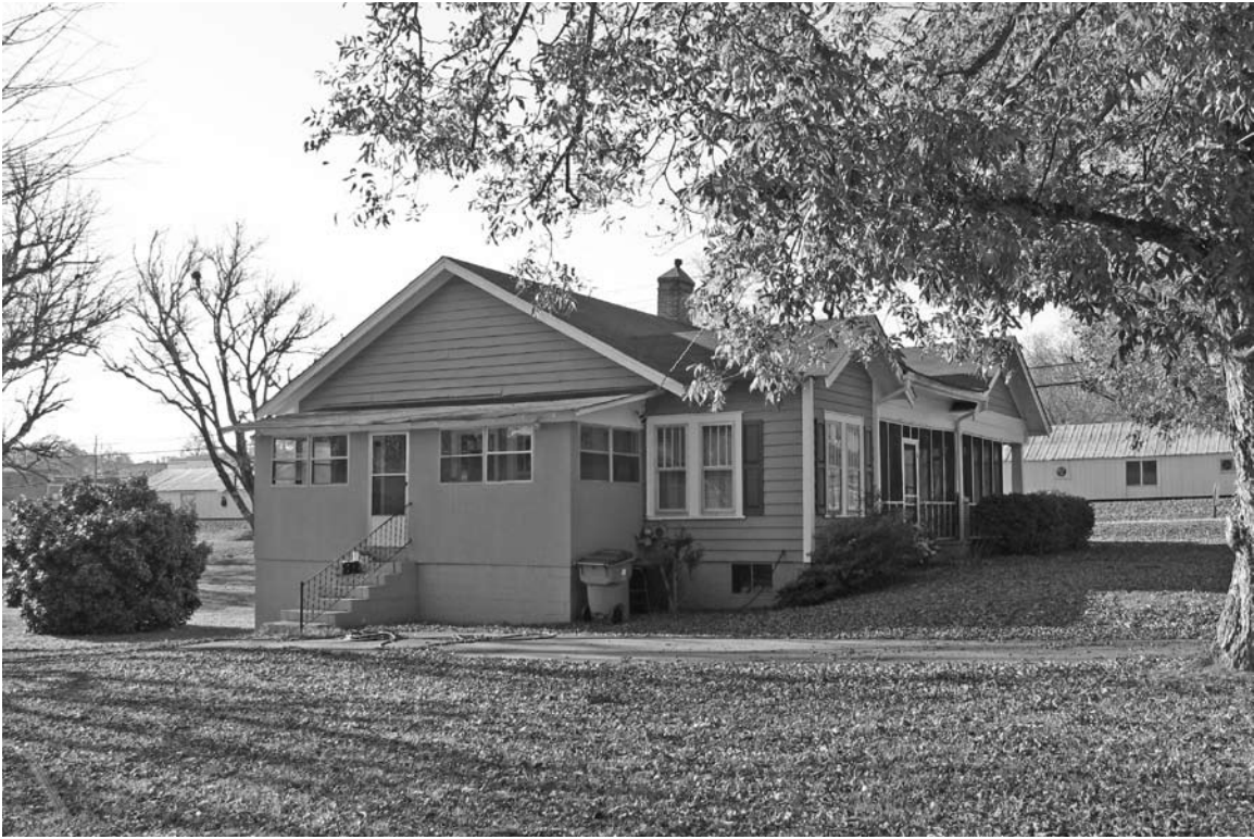
Photograph 3: View of the rear elevation of the resource.
