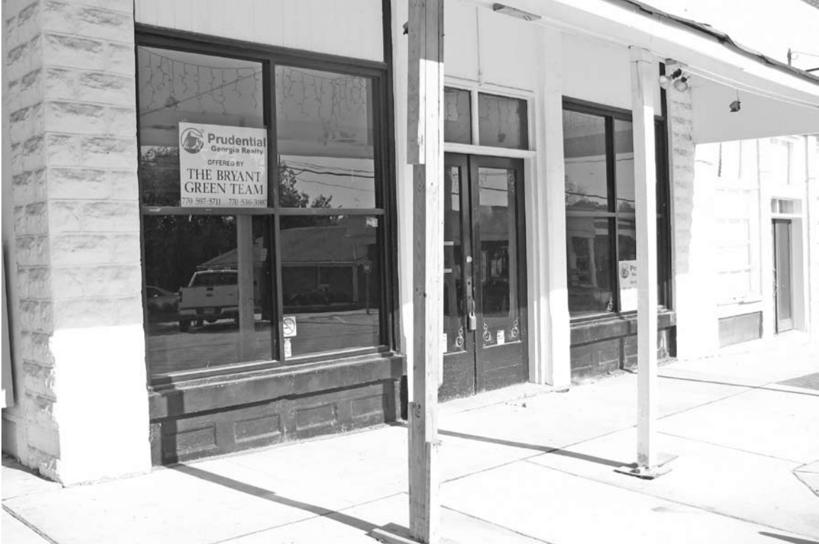
Photograph 4: View looking at the front elevation of the resource.
