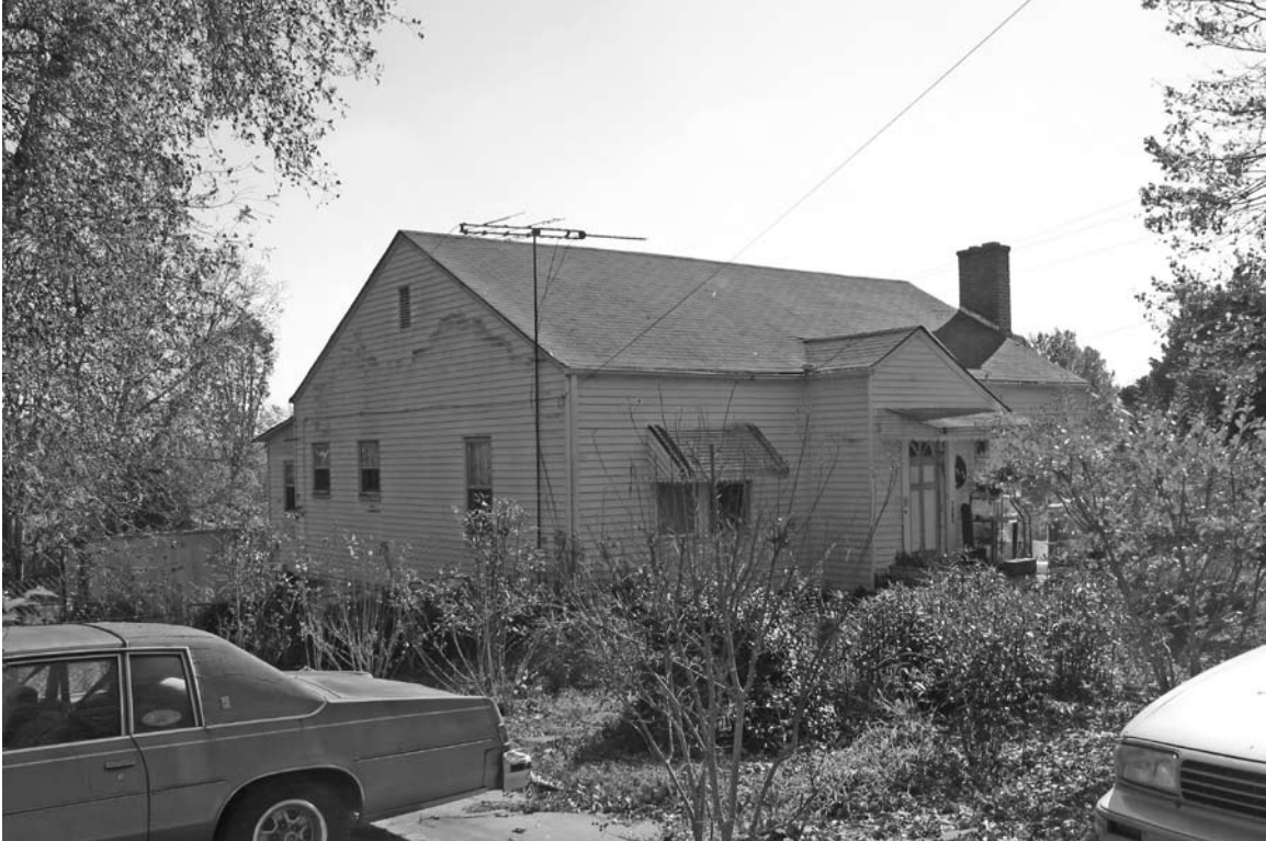
Photograph 2: Left elevation of the resource.
