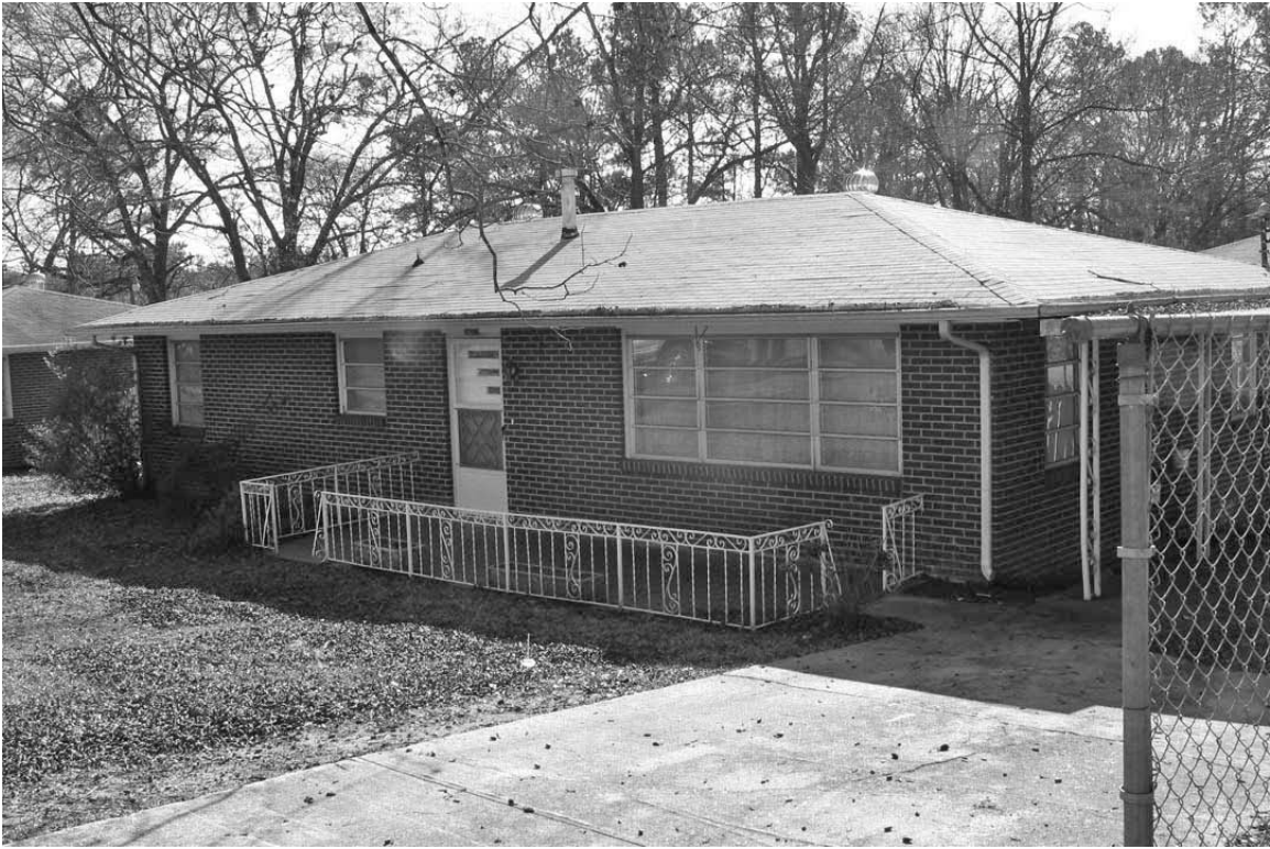
Photograph 1: View looking at the front elevation of the resource.
