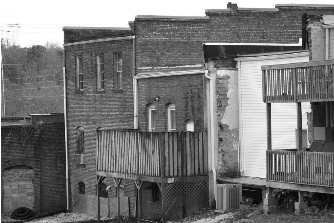
Photograph 2: Rear elevation of the resource.
