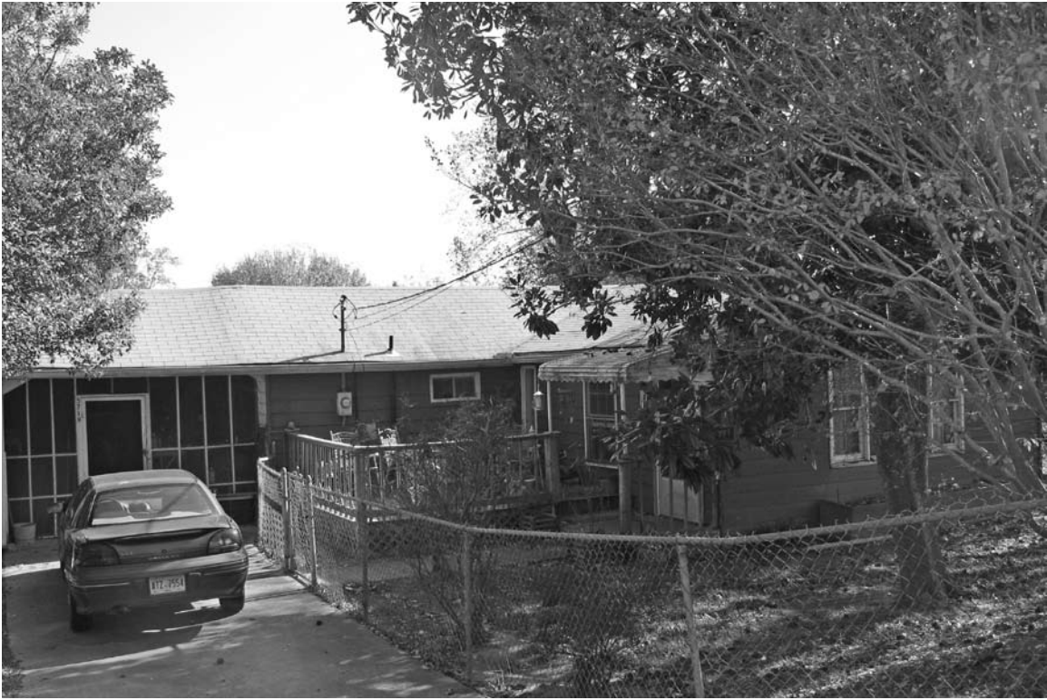
Photograph 3: View looking at the front elevation of the resource.
