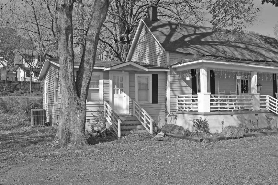
Photograph 2: View of the front left side of the resource.
