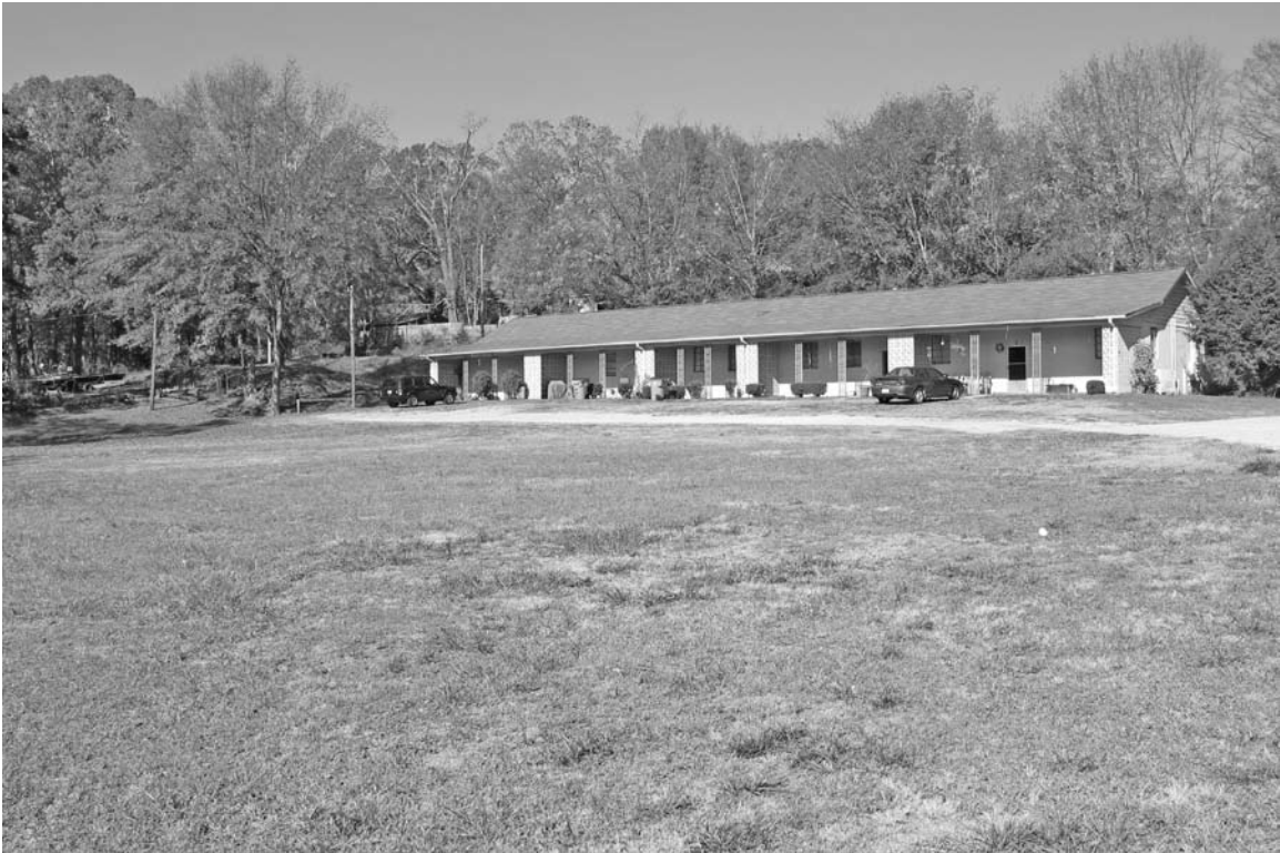
Photograph 3: View looking at the outbuilding.
