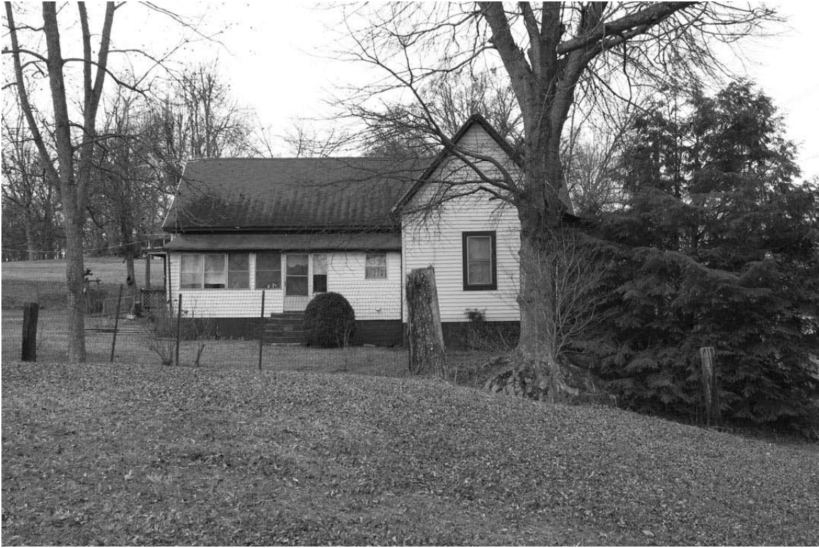
Photograph 3: View looking at the left side elevation of the resource.
