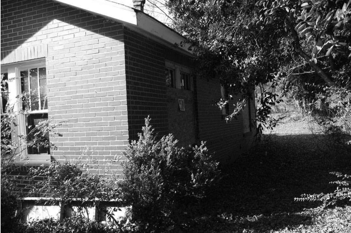
Photograph 4: View looking at the right side and front elevation of the resource.
