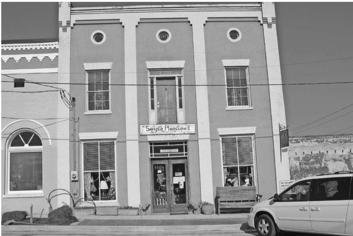
Photograph 1: Front elevation of the resource.
