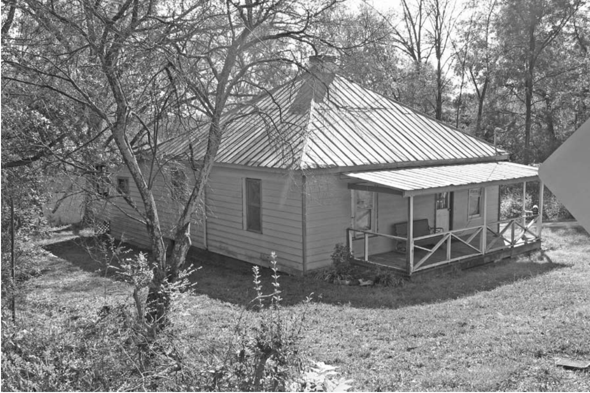
Photograph 1: View left side elevation of the resource.
