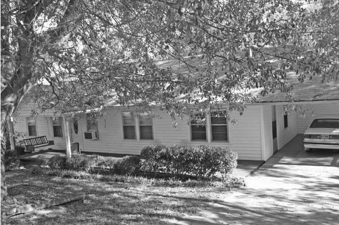
Photograph 4: View of the front and right side elevation of the resource.
