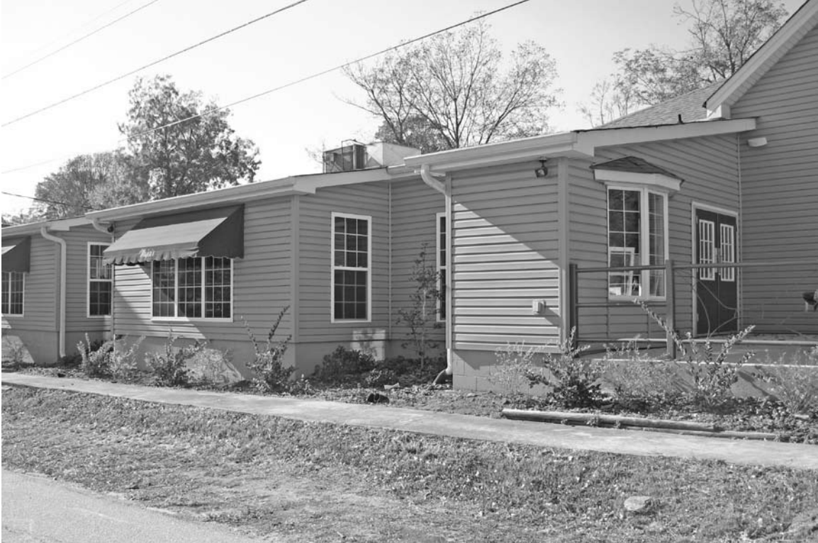
Photograph 4: View looking at the left side elevation of the resource.
