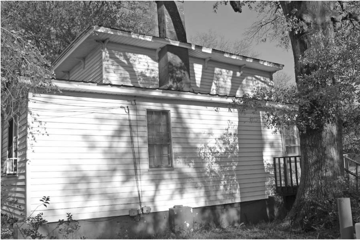
Photograph 3: View looking at the rear portion of the left elevation of the resource.
