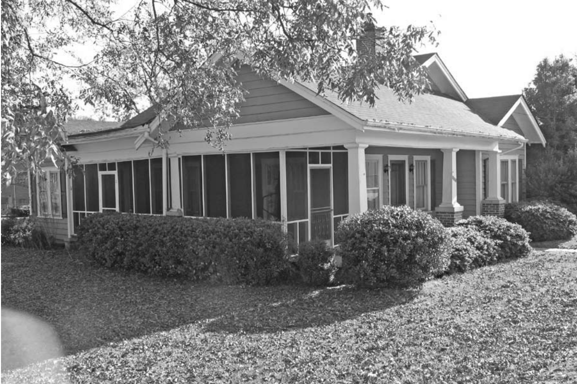
Photograph 2: View looking at the front and left side elevation of the resource.
