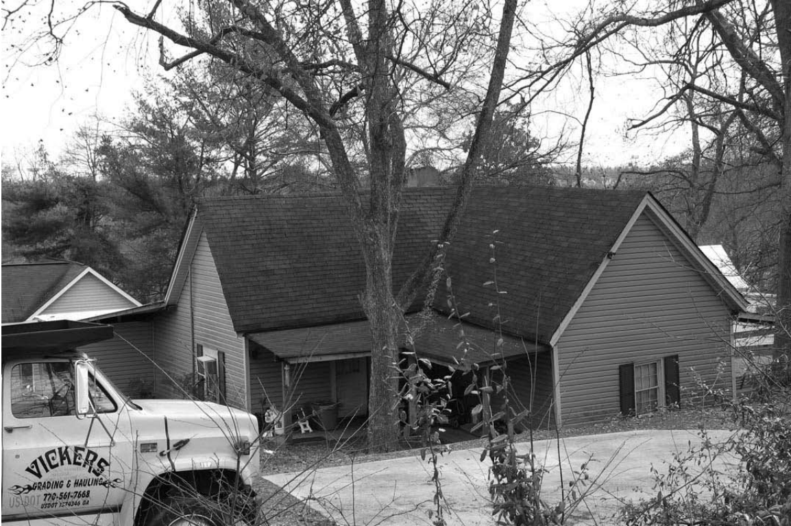
Photograph 4: View looking at the right side and rear elevation of the resource.
