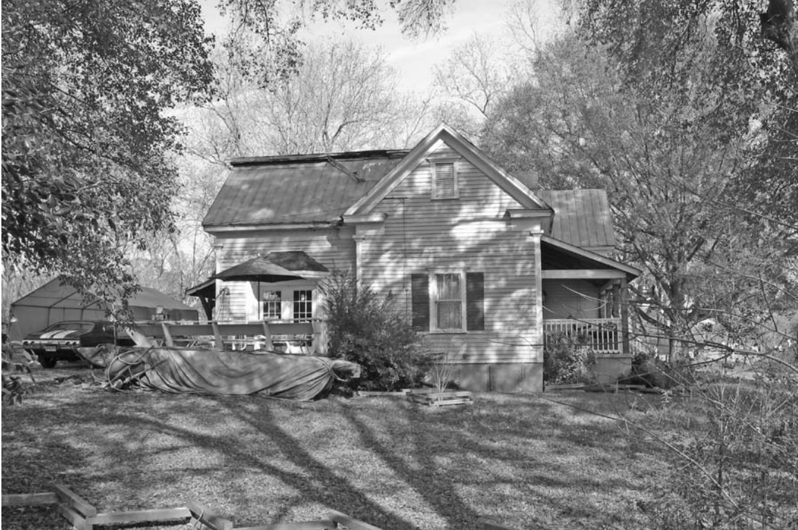
Photograph 2: View looking at the left side elevation of the resource.
