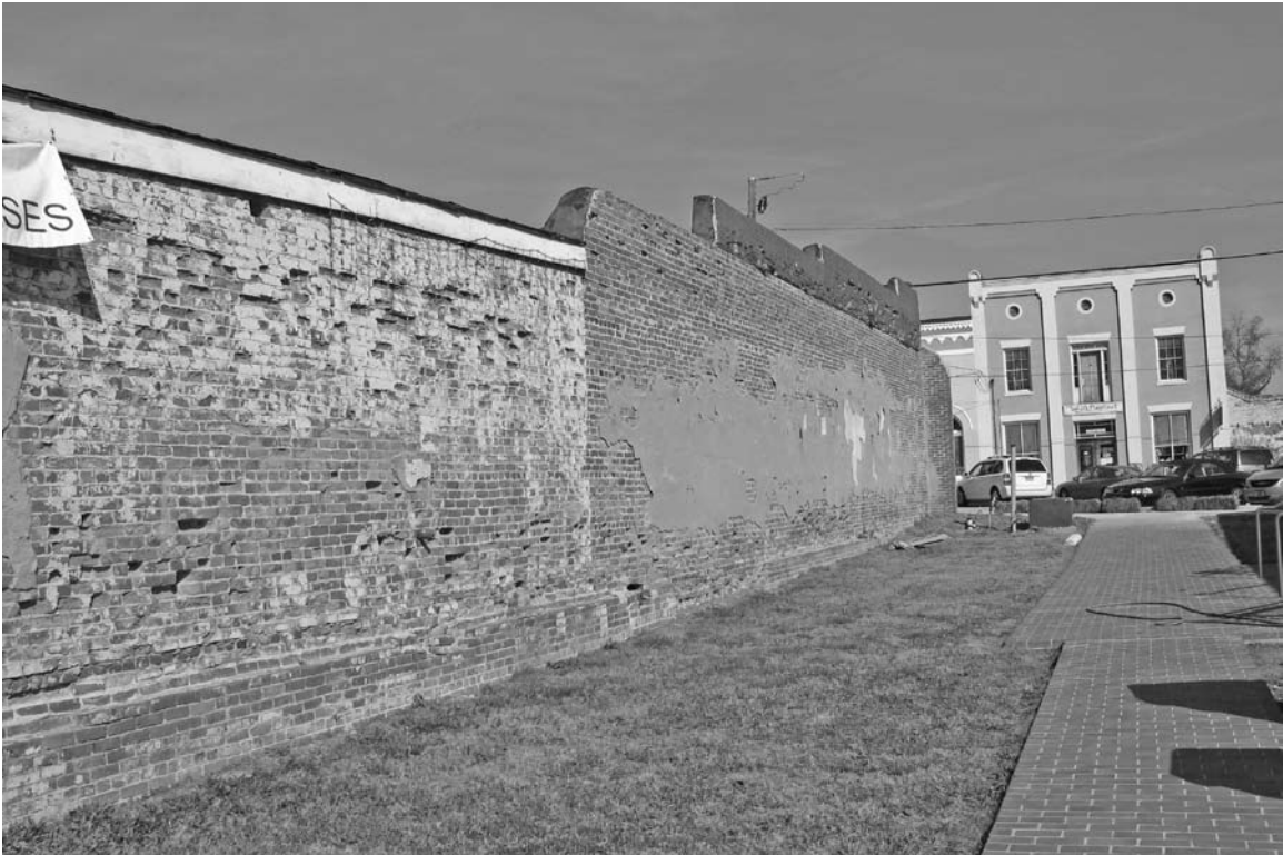
Photograph 3: View looking at the left side elevation the resource.
