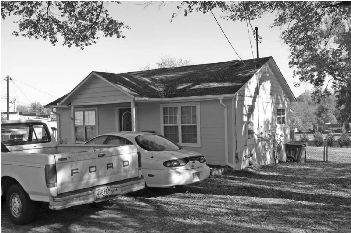
Photograph 3: View looking at the right side elevation of the resource.
