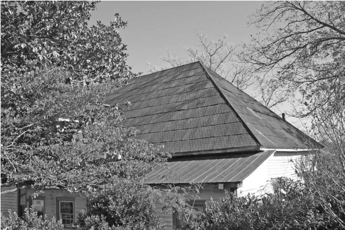
Photograph 1: View looking at the roof of the resource.
