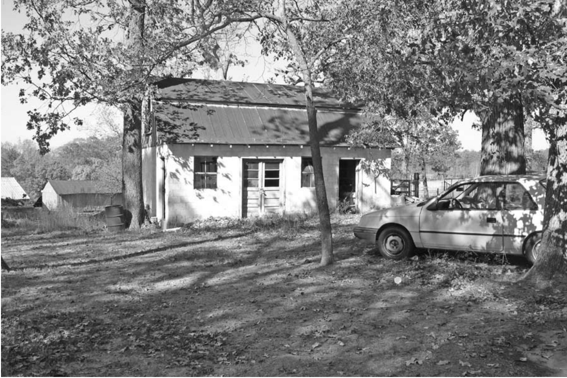
Photograph 5: View of outbuilding to the rear of the resource.
