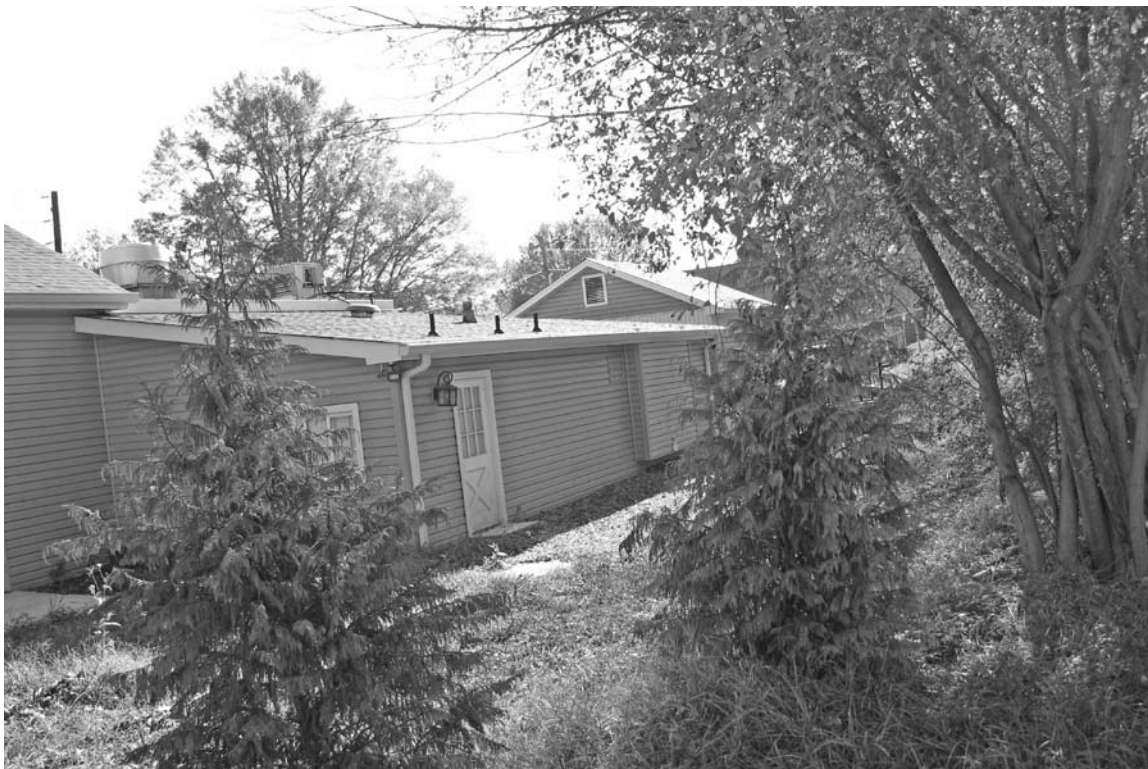
Photograph 1: View looking at the rear elevation of the resource.
