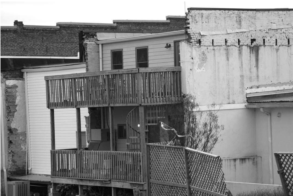
Photograph 2: Rear elevation of the resource.
