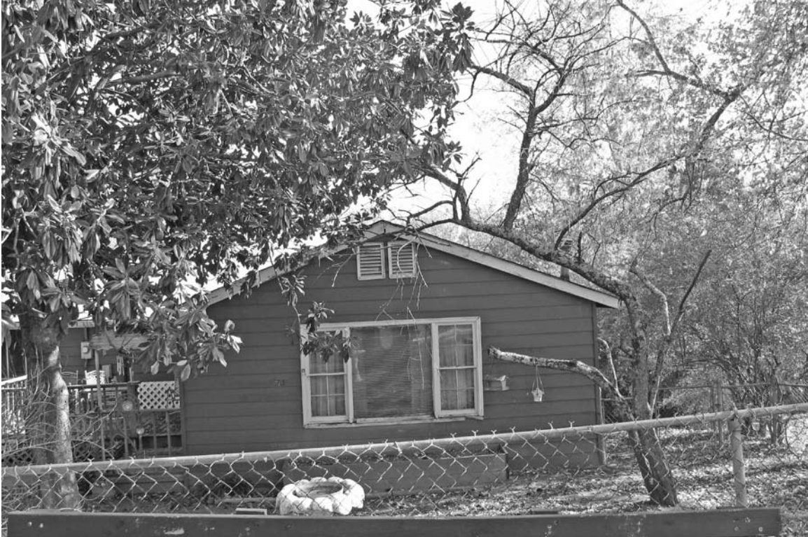
Photograph 2: View looking at the front elevation of the resource.
