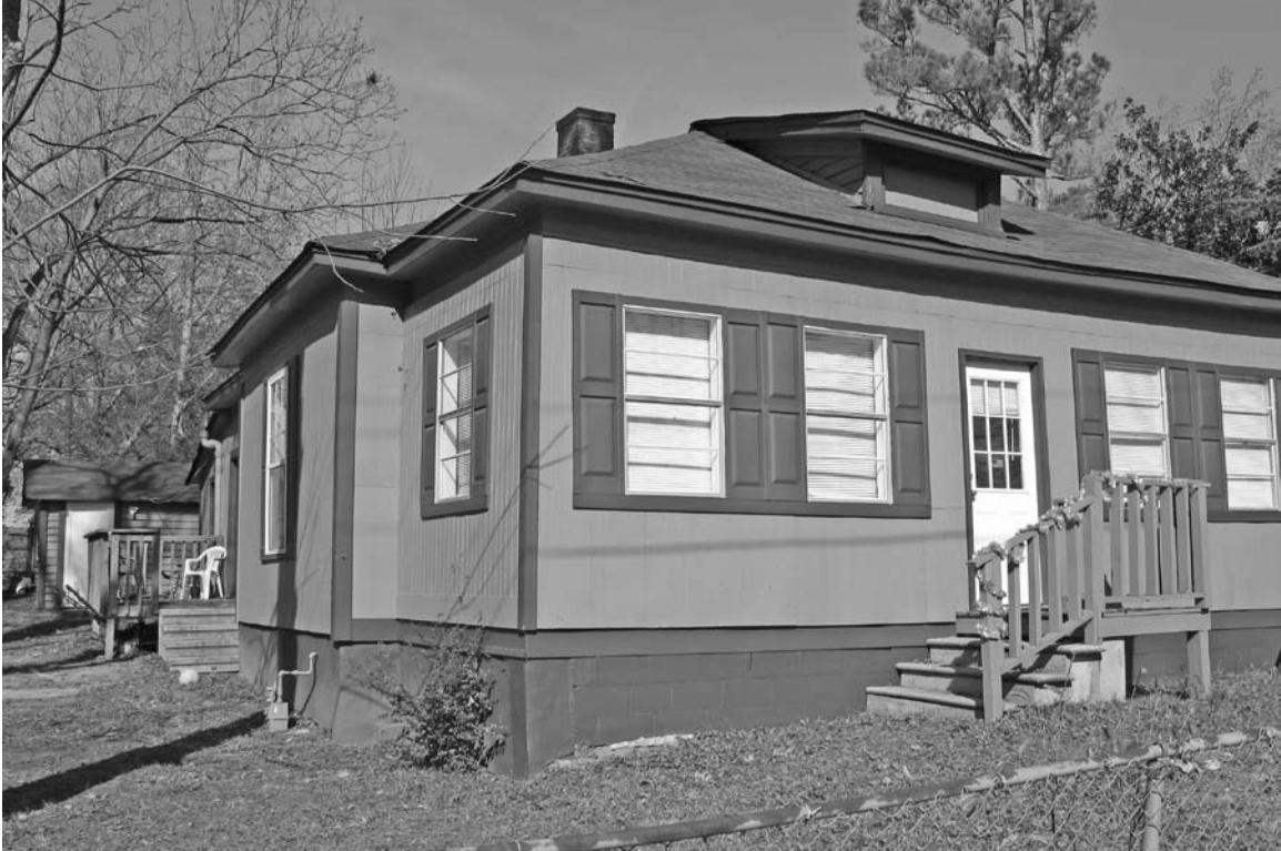
Photograph 2: View looking at the left and rear elevation of the resource.
