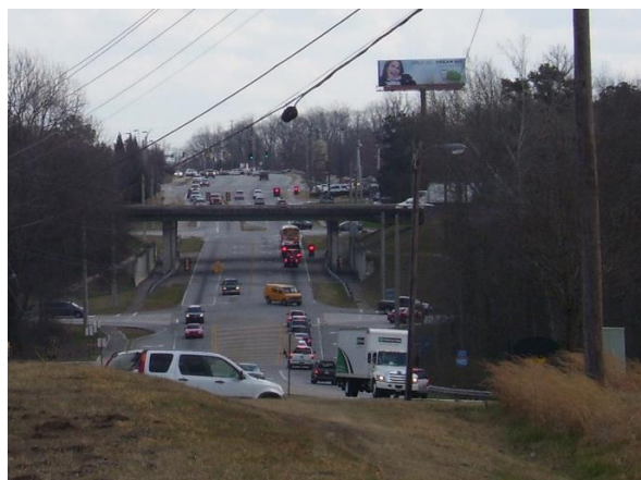
A view of Phil Neikro Boulevard/ Spout Springs Road eastbound under Interstate 985 (bridge) (Thurmon Tanner Road is in the forefront)
