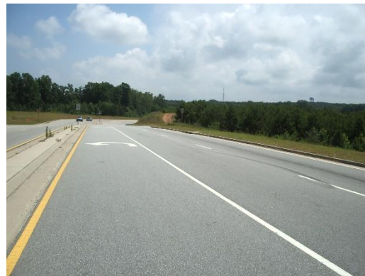
Thurmon Tanner Pkwy. Northbound from Phil Neikro Blvd.
