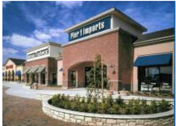
Well Articulated Buildings with Pitched Roofs and Canopies or Awnings
